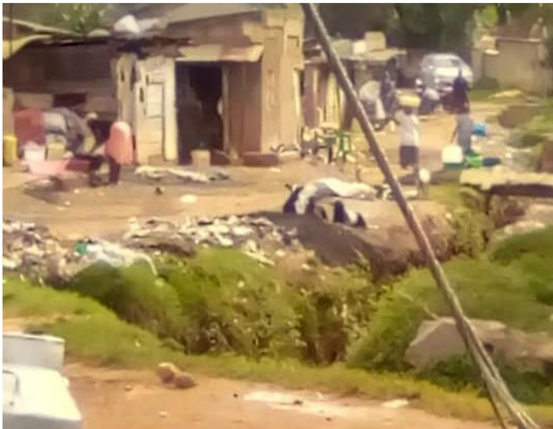
Figure 2: Drainage turned into a refuse collection site
